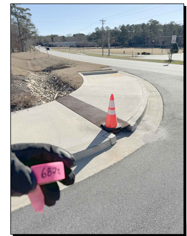
① → FLUME (METAL COVER) ② → FLARED END SECTION
