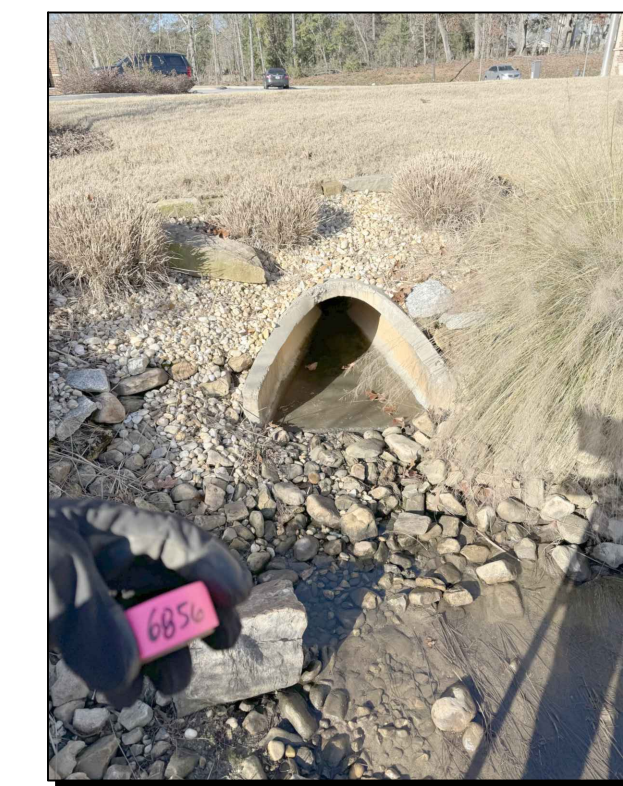
① → FLUME (METAL COVER) ② → FLARED END SECTION
